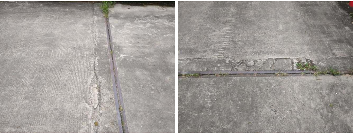
0#桥台接坡破损
