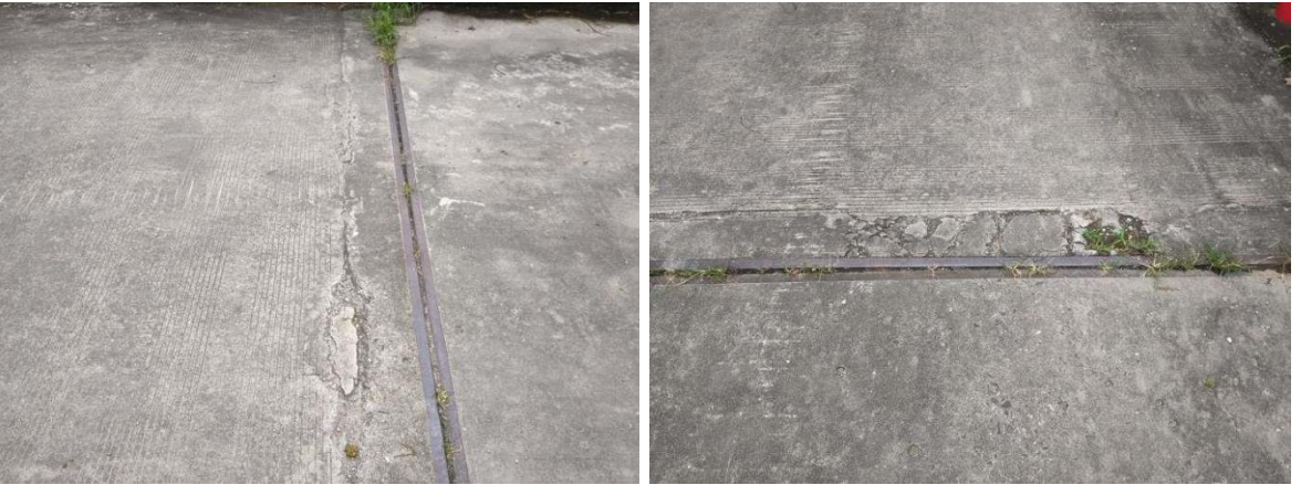
0#桥台接坡破损
