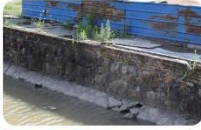
堤岸破损、裂缝
